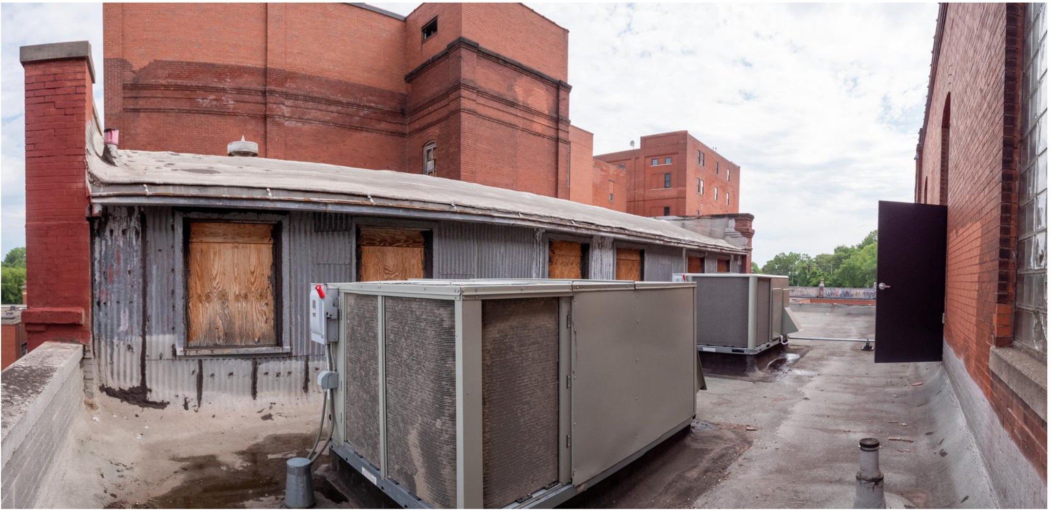
Above: the rooftop exterior – Historic Hamms Brewery.
